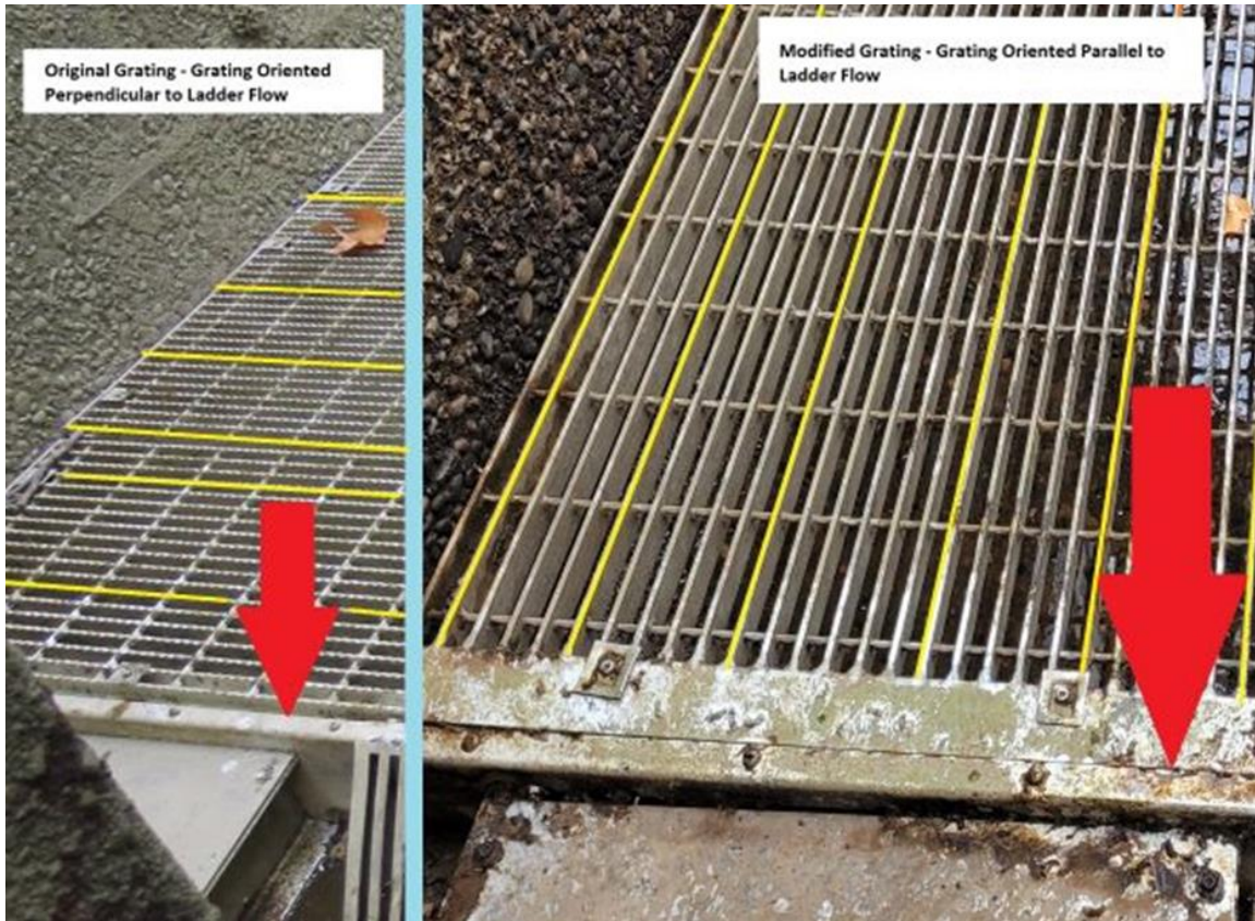
Figure 6: SFL LTS grating The red arrow indicates the entrance to the lamprey trap, and the yellow line indicates the grating orientation.
